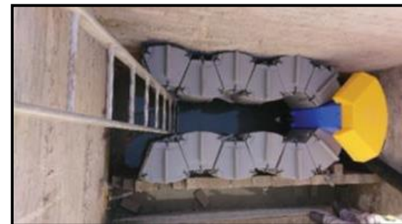
Figure 3: Up-Flow Filter installation.
